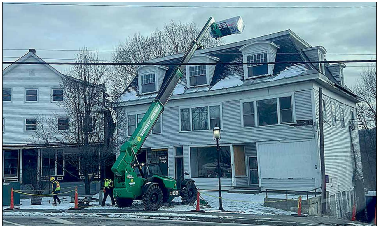
Another vacant building in Hillsborough's Central Square is being completely renovated.
