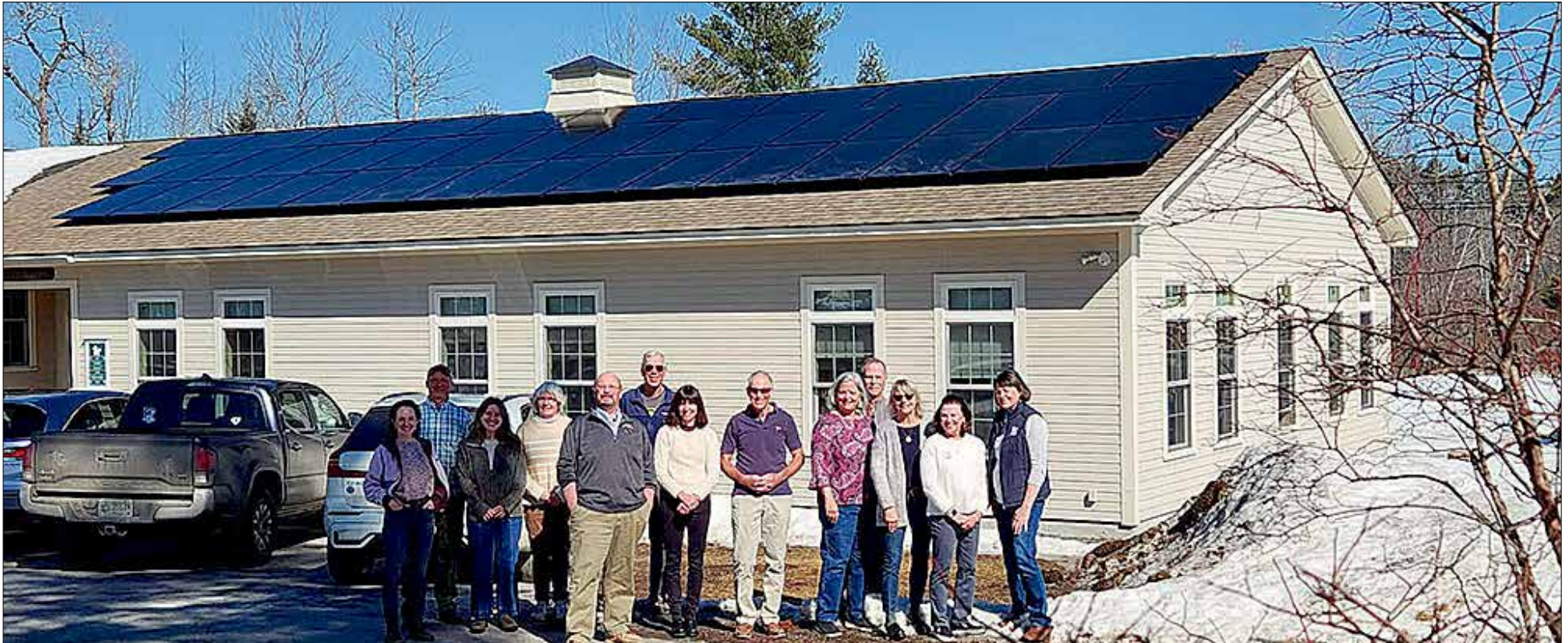
Thanks to a gift from Lisa and Jamie Hess of New London, the Ausbon Sargent office building on Pleasant Street is now solar powered.
