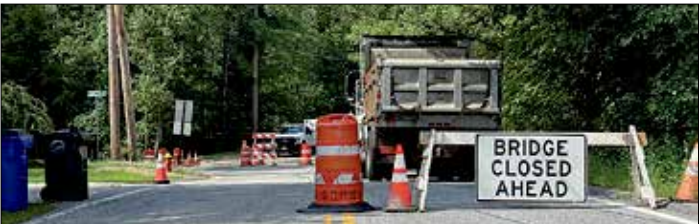
Construction on Goffstown's Henry Bridge Road is moving along as intended and is targeted for completion by the end of the month.
